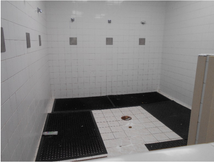
Lincoln Living Unit – Bathroom shower area
