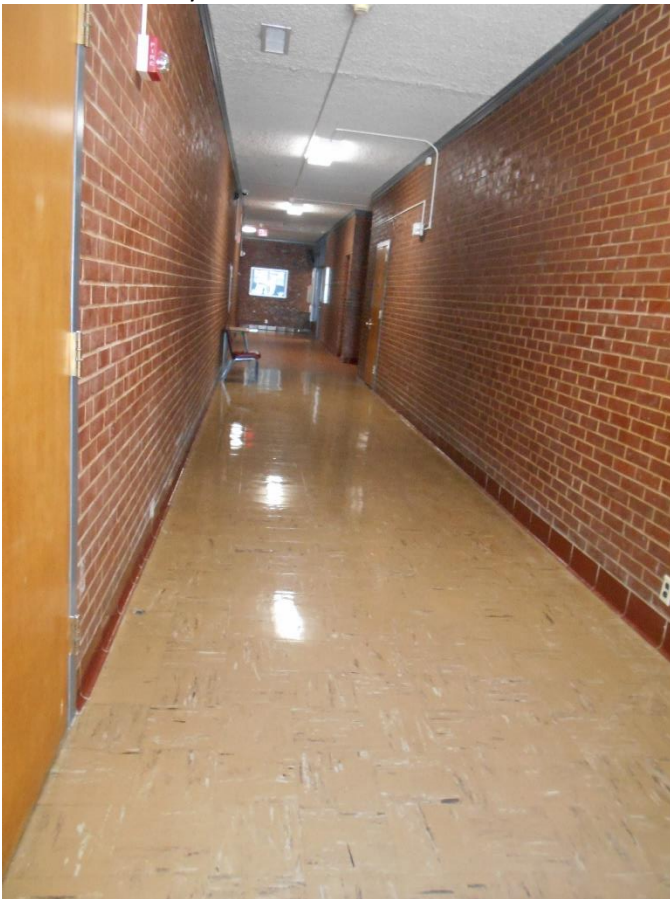
School – hallway from south outside door to office area
