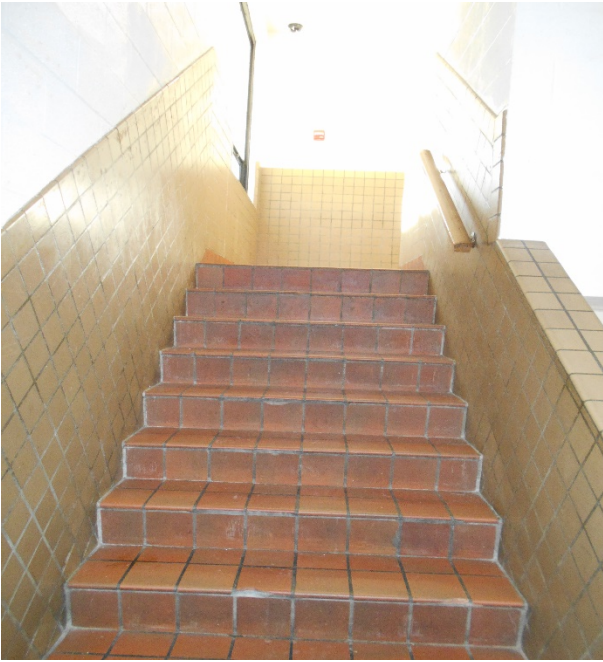
Lincoln Living Unit – Stairs to second floor (2 flights)
