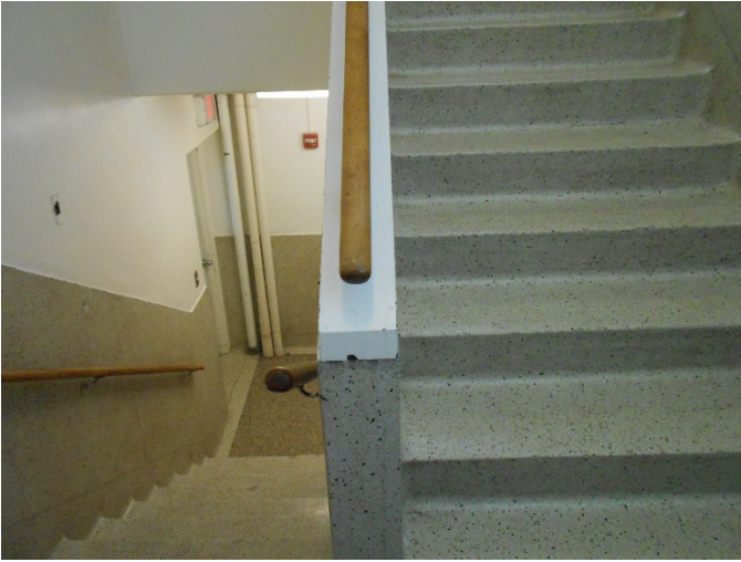
Morton Living Unit – stairs to second floor
